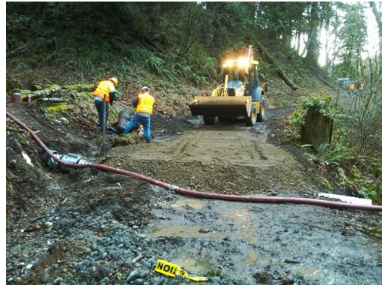
Backfilling the replacement drainage culvert above the area of trail washout.
